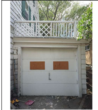
Above: The garage on the north side of the house that will be demolished. 09/12/2019
