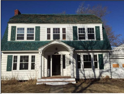
Above: The front (east) of the house. Note the garage on the north side. 09/12/2019
